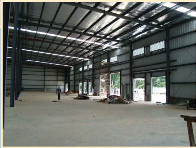
Building I – facade and interior finishes are underway
