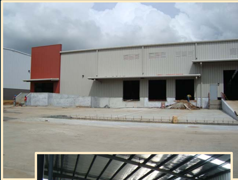
Warehouse Building I
