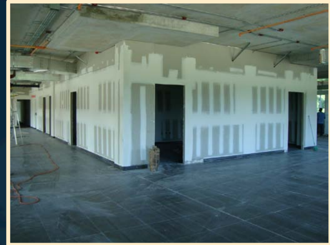
New tenants as VF Corp continue with their interior improvements
